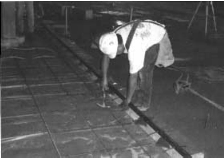
Left: the plate dowel pocket former is nailed to the form prior to casting the first slab.
