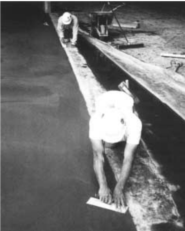
Above: Additional reinforcement in column detailing provides protection against re-entrant cracking. Left: Hand troweling of the joints ensures that the joints are flat.
