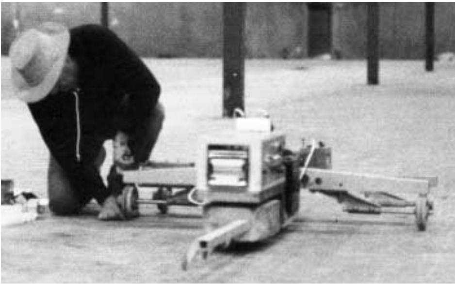
When cracking compliance of the superflat slabs, the Profileograph wheels are set to match the wheelbase of the forklifts that will operate in the warehouse.
